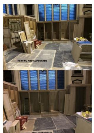
The construction of the new WC has progressed well, the walls have been fully constructed and much of the pipework is now in place. Ducts through the south wall for the extractor fan and a separate vent have been created and if you look carefully on the outside of the south wall between the south porch and the west end of the church, you'll see where these come out.
