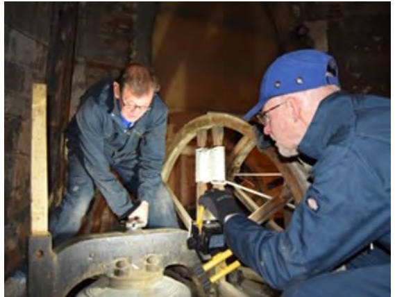
Bell ringers re-installing the clappers
