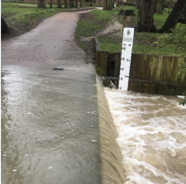
The flooded bridge by Bridge End Gardens.
